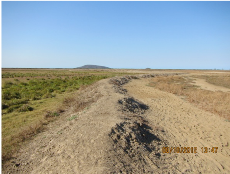
Figure 10. The removal of bunds such as this, can facilitate saltmarsh repair. Source: GBRMPA
