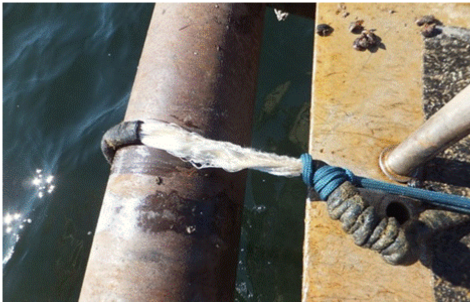
Figure 4-9 Degloved strop of the Maple 42 mooring during servicing.
