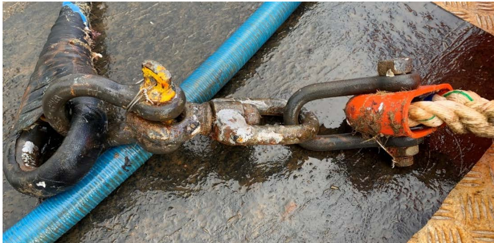
Figure 4-5 Mild galvanic corrosion of the hardware set on the Roberts 36 following cleaning
