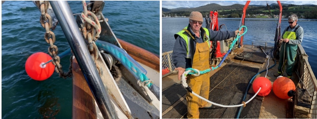
Figure 4-5 a) replacement of the Nylon with polypropylene b) new chaffing protection solution. Mr Bob Kelly (left) and Mr Jeff Whyman from Channel Mooring Maintenance.
